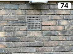
Air Brick (6XLYNF) Inspection Type: Visual
